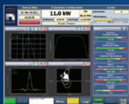
AUI Control System
