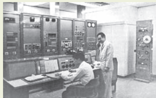
Radio Hong Kong's Broadcasting Centre (1969)
