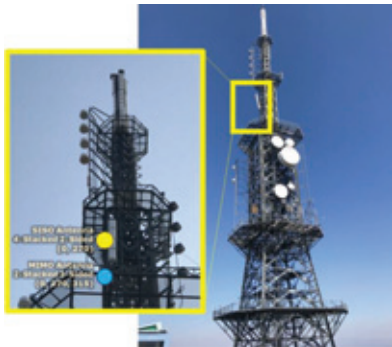
Antenna installation on a transmission tower: SISO (top) and MIMO (bottom)
